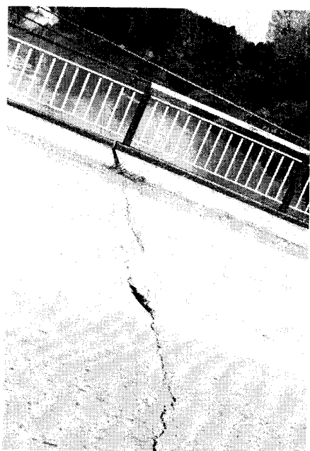
Figure 2 Typical failure of buried joint
